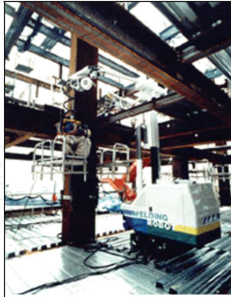
Fig. 11. WR mobile robot for column welding
