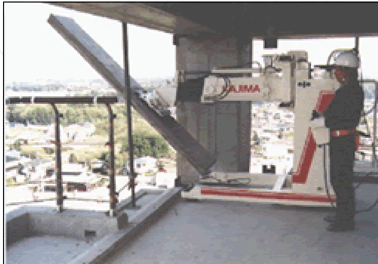
Fig. 7. Kajima's interior wall assembly robot
