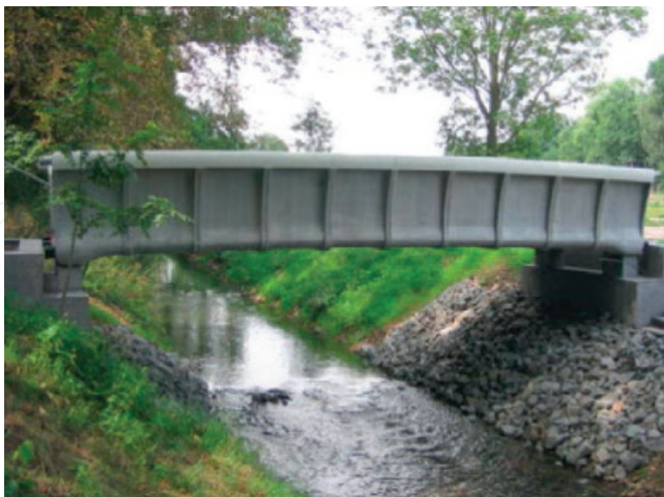
Figure 12. First segmental TRC Bridge in Oschatz, Germany [94].
