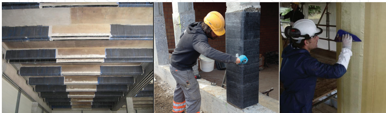
Figure 14. Strengthening of existing concrete structural members using unidirectional carbon and aramid sheets [98].
