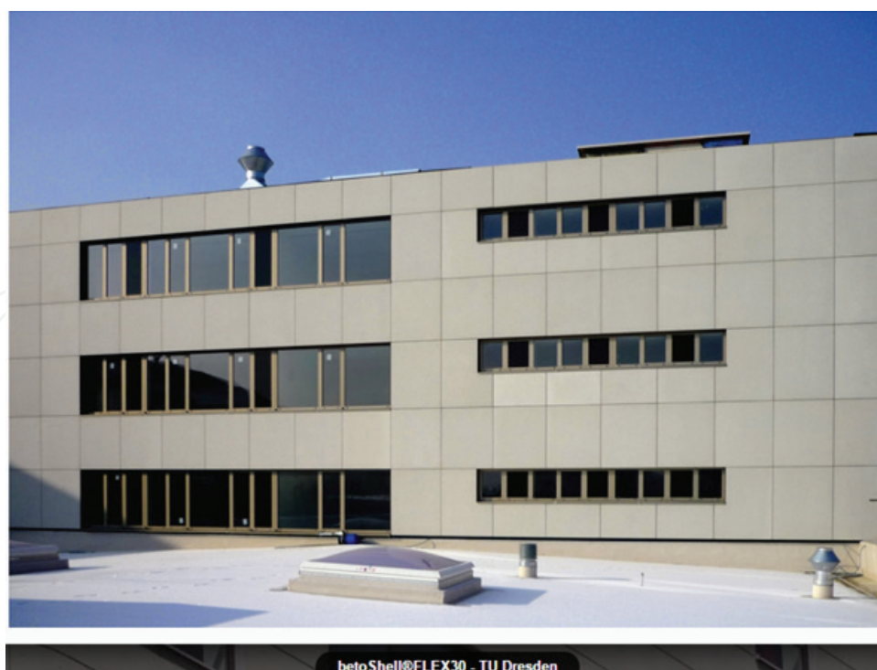
Figure 13. бетоShell© façade application developed by Hering Bau [95].
