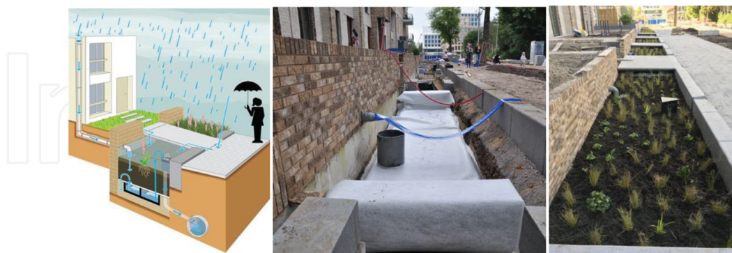
Figure 4. Left to right: Schematic of the green stream system, under construction and on the day of completion.
