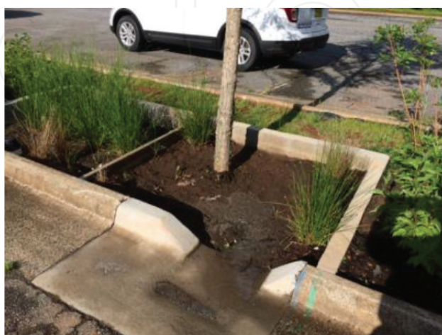
Figure 6. A tree pit receiving urban sediment from an adjacent parking area, Greensborough, North Carolina, USA.
