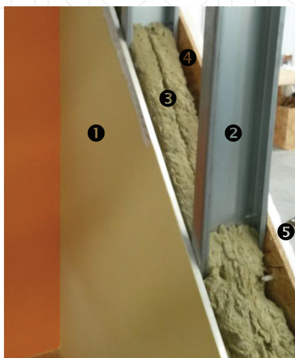
Figure 2. Materials in a LSF wall crosssection [30]. Legend: Gypsum plaster board; Cold-formed steel profiles; Mineral wool; OSB; and ETICS with EPS.
