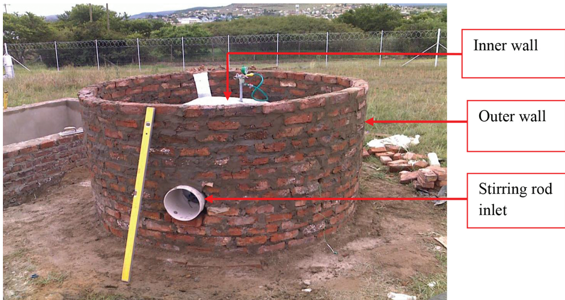
Figure 7. Constructed second wall of the biogas digester.
