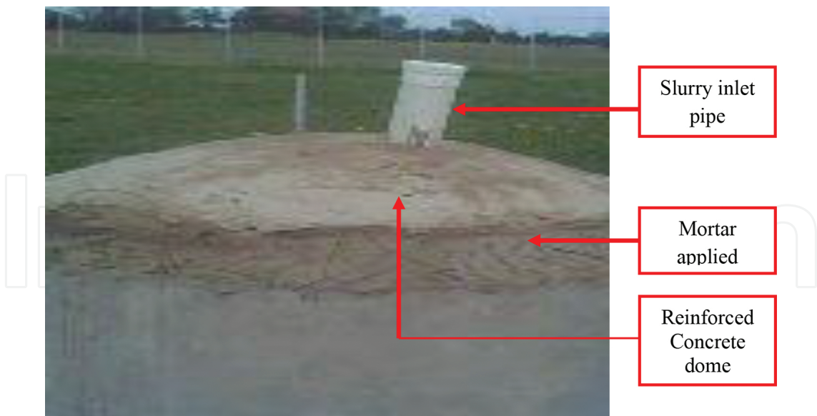
Figure 6. Biogas digester with a reinforced concrete dome.
