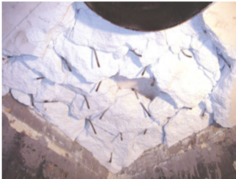
Figure 12. The part of the combustion zone structure in the heating unit used in oil refineries damaged by explosive spalling (metal anchors can be seen on the photograph) [29].
