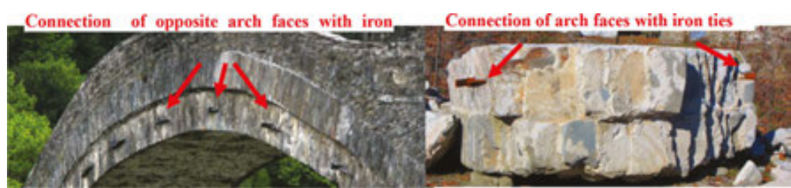
Figure 12. Iron ties used to connect the two opposite faces of the primary arch in Plaka Bridge.
