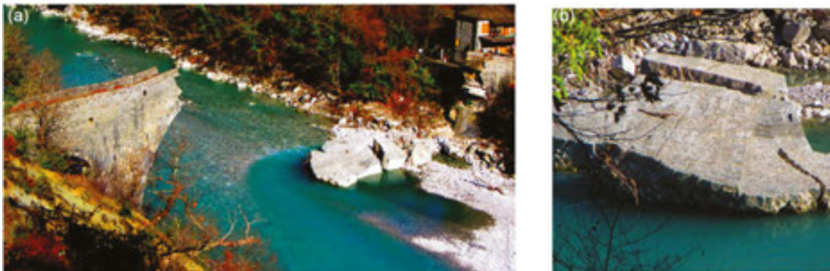
Figure 50. (a) View of the Plaka Bridge after the collapse from the West bank. Note the total destruction of the mid-pier (see also Figure 7d ). (b) Close-up of the total destruction of the mid-pier of Plaka Bridge (see also Figure 7d ).
