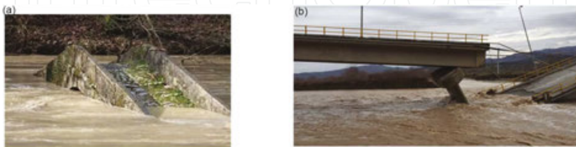
Figure 49. (a) Almost total flooding of a stone masonry bridge and (b) tilting of a mid-pier and partial collapse of the Diava-Kalampana reinforced concrete bridge in Thessaly, Greece (16th January, 2016).
