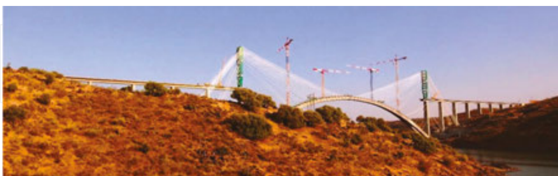
Figure 27. Arch bridge erection by cable-stayed supports at sunset, Estremadura, 2015.
