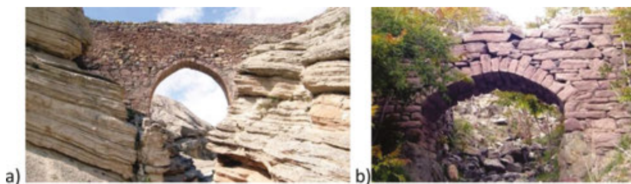
Figure 10. Stone arch bridges in the vicinity of Sille Village near Konya: (a) double parabolic arch structure; (b) parabolic arch with the deck partially ruined.
