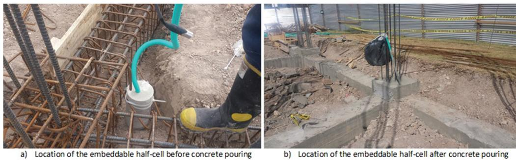
Figure 9. Installation of the embeddable half-cell.
