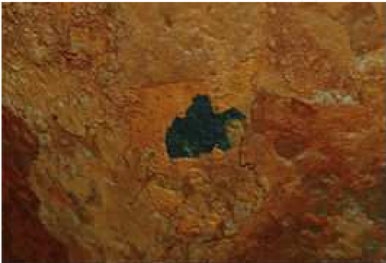
Figure 1. Accelerated Low Water Corrosion Observed on Steel Piles above Water during Spring Tide [2]
