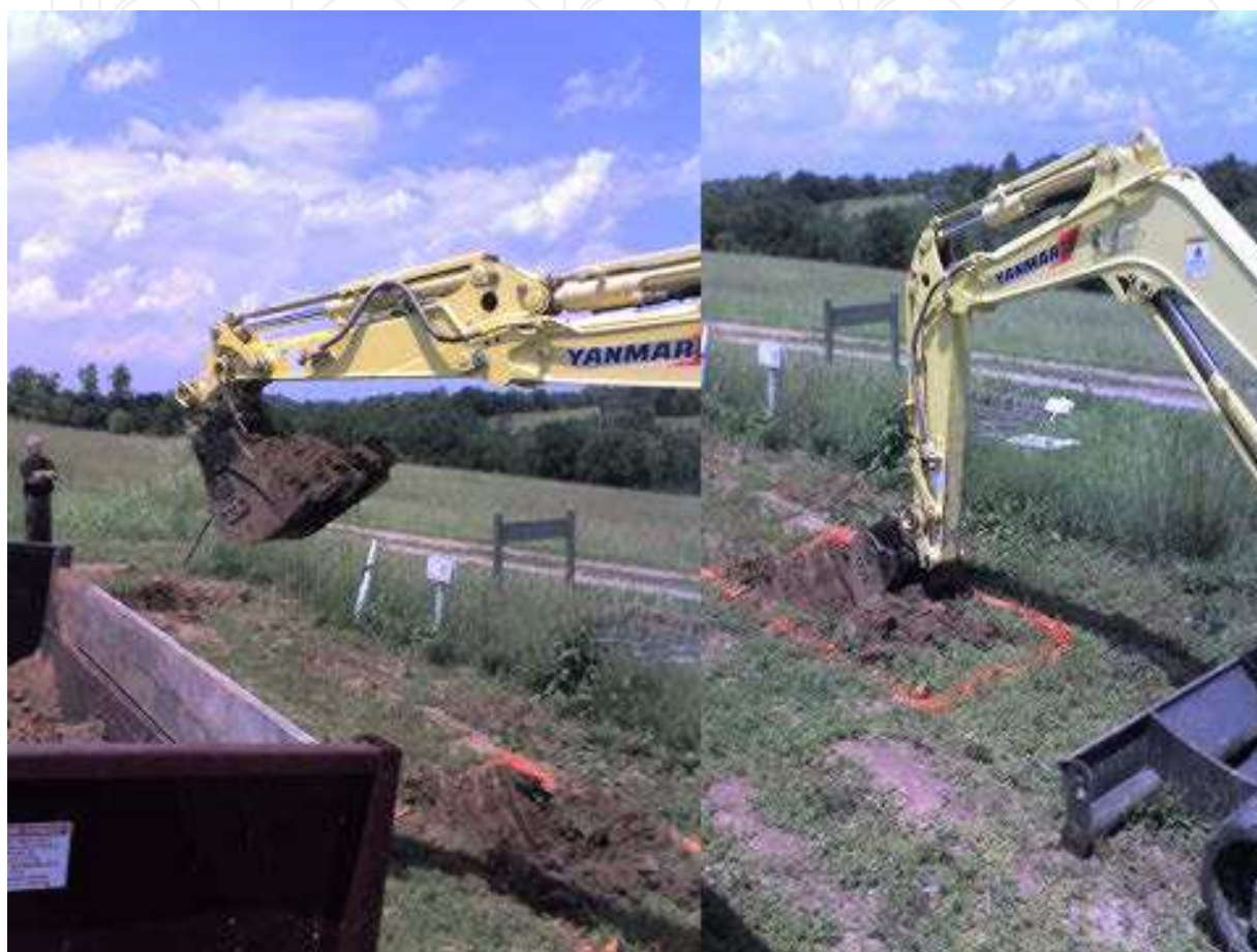
Figure 7. Preparation of soil cavity for biofilter installation at Kentucky State University (Franklin Connty, KY) for trapping herbicides residues in surface runoff water.
