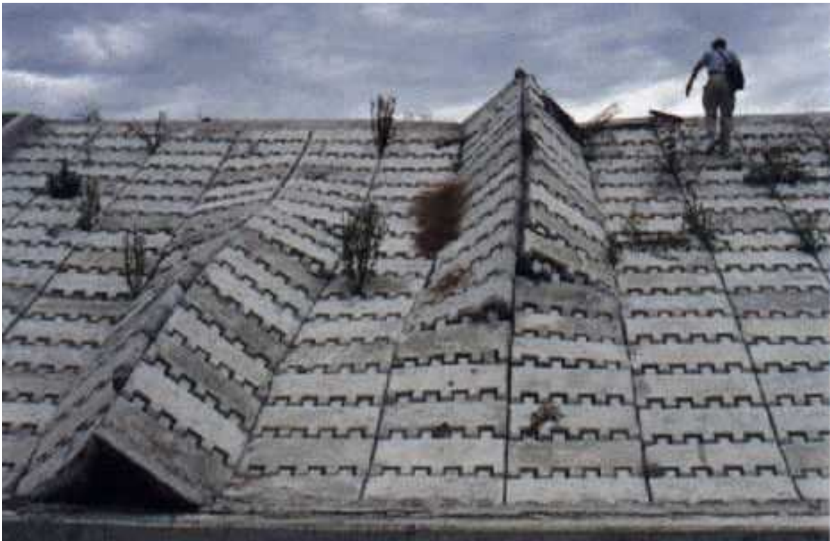
Figure 1. Buckling of river embankment lining after the 1999 Chi-Chi earthquake [32]
