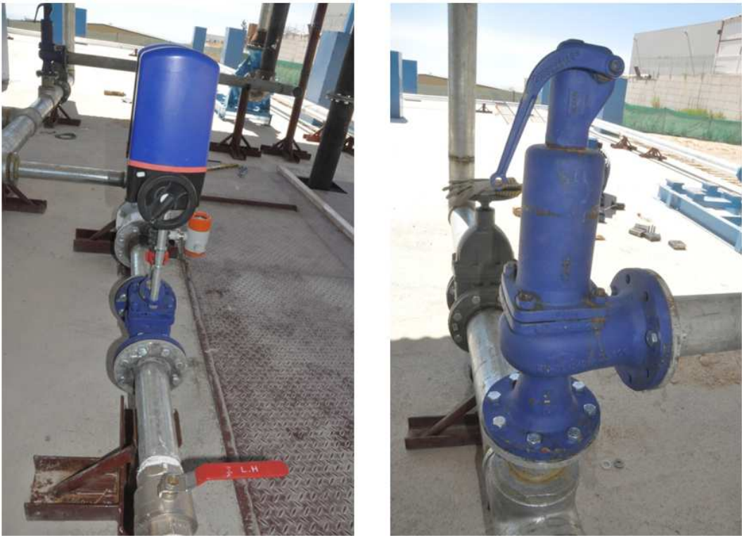
Figure 9. Analog valve (left) and pressure relief valve (right)
