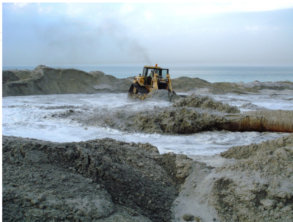
Figure 2. Sand and mud materials are pumped from a marine burrow area into the reclamation site. ‘Dyar Al Muharraq’ development in Bahrain (2013).
