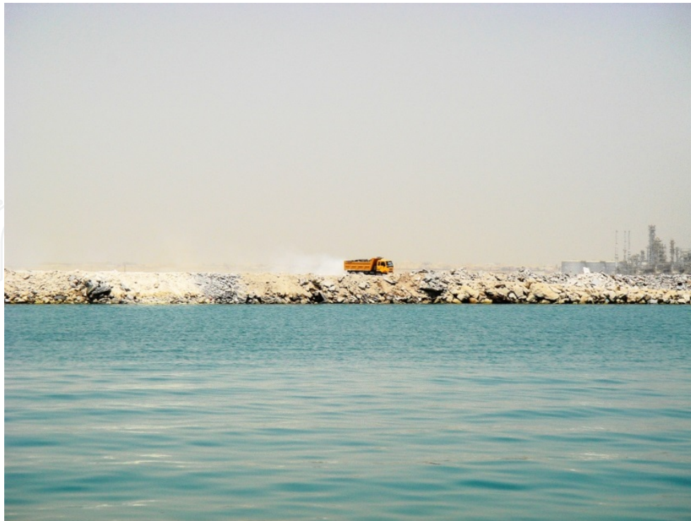
Figure 3. Rocks and sands extracted from nearby quarries are used to reclaim a coastal area along the eastern coastline of Bahrain (2012).
