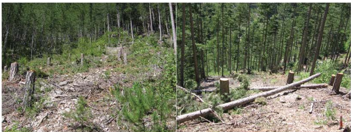
Figure 34. Examples high stumps and felled trees diagonally to the direct slope and anchored on high stumps in the case study Val Drôme
