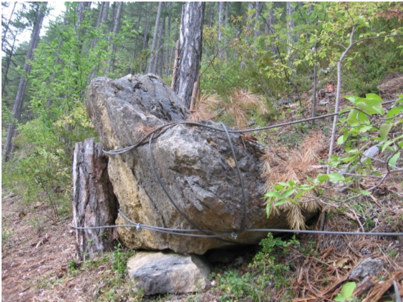
Figure 38. Example of anchorage of an unstable deposit rock in the Val Drôme case study.
