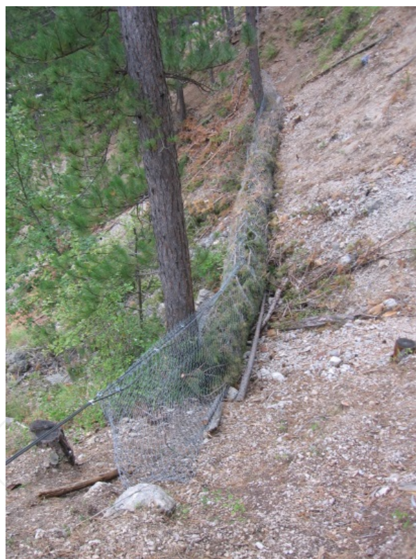
Figure 36. Example of use of a Fasnet eco-engineering work in the case study Val Drôme
