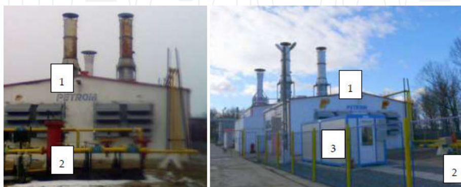
Figure 4. Control – measurement station for natural gas at 2xST 18 – Suplacu de Barcău plant (left) with booster (right) 1 – cogeneration power plant; 2 – control – measurement station; 3 – booster
