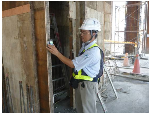
Figure 5. Displayed safety staff used RFID-enable smartphone to scan RFID tag. (A)
