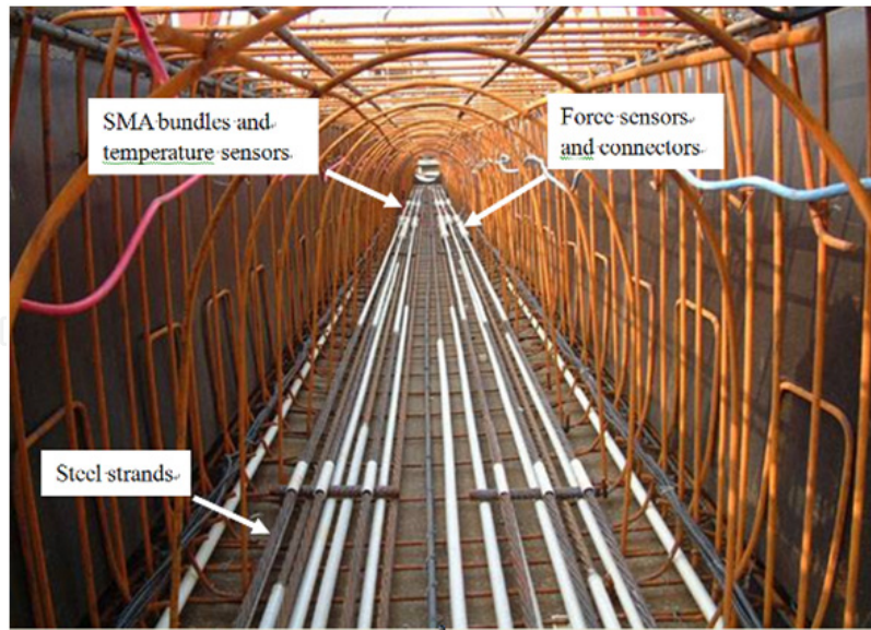
Figure 32. Framework of steel reinforcement with stretched SMA bundles
