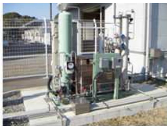
Figure 12. The adsorptive, isolated methane concentrating device
