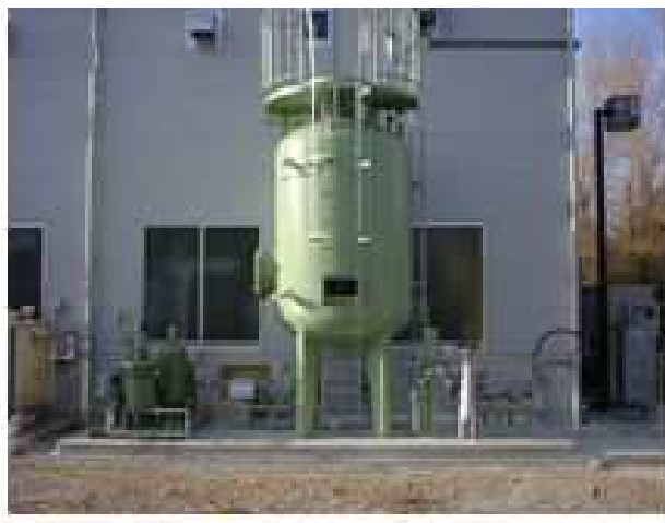
Figure 10. The adsorptive biogas storage system
