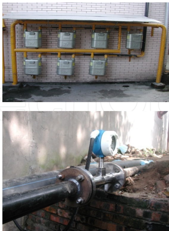
Figure 12. One MEMS meter can replace seven diaphragm meters with better accuracy.
