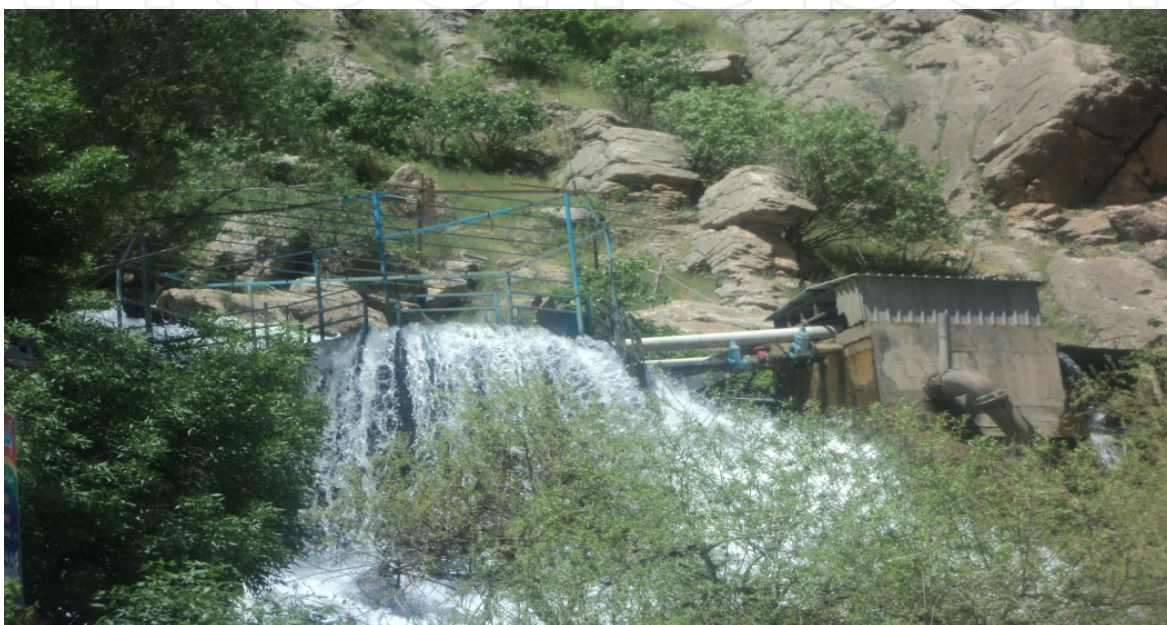
Figure 17. Shows the intake and the penstock (pipeline) of Bekal water treatment plant
