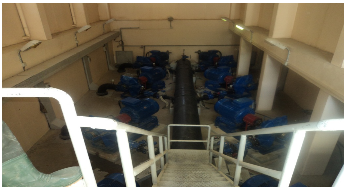
Figure 18. Shows the high head pump station
