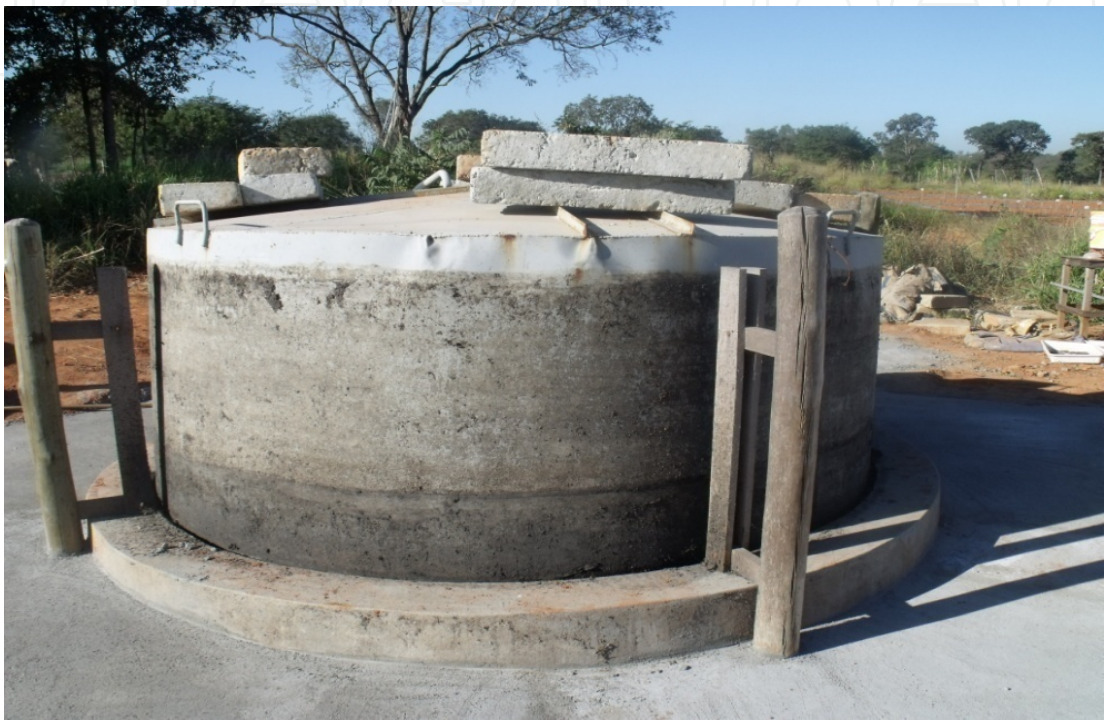
Figure 3. Biodigester Indian Model.
