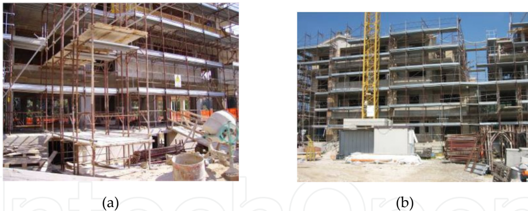
Figure 5. Typical conditions of a construction site in an advanced construction phase, (a) just after the structural frame completion and (b) after the construction of the envelope and of the internal partitions.
