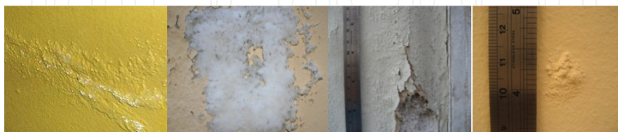
Figure 11. Swelling, efflorescence, cracking and blistering (Moura, 2008).
