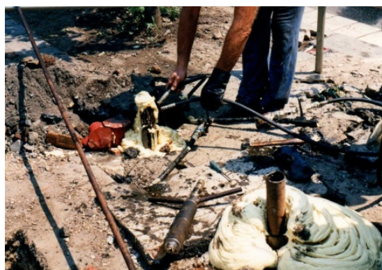
Figure 23. Sealing of the borehole with PU grouting
