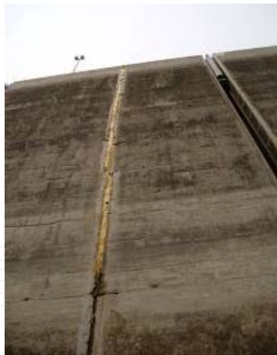
Figure 30. Dilatation joint after the grouting
