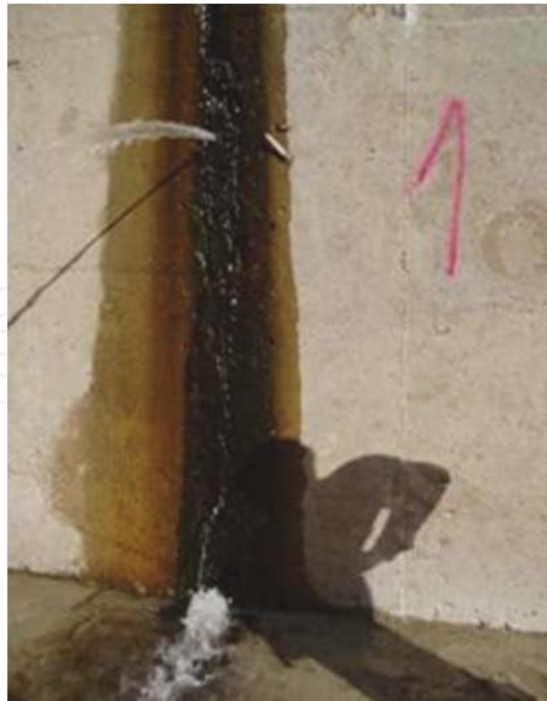
Figure 29. Dilatation joint before the grouting
