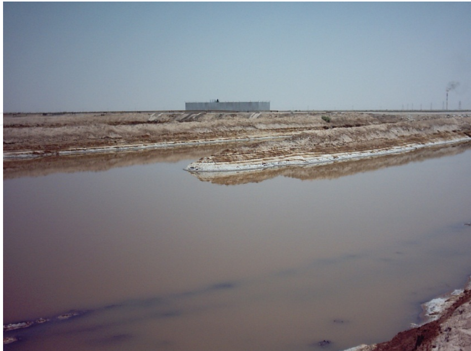
Figure 4. Mud pit condition after drilling operation.
