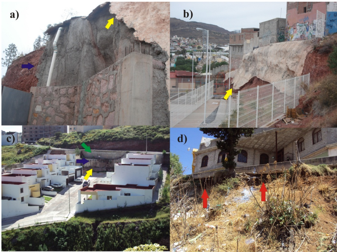
Figure 2. Images showing the erosion hazards associated with different lithology: a) and b) are in the granitic facies of the Zacatecas Conglomerate; c) moderately consolidated facies of the Conglomerate; and d) deformed lava flows from Las Pilas Complex. Yellow arrows point toward the first attempt of damage repair. Purple arrows are the sites where a second repair phase has been attempted; while the green arrow shows a third repair phase. The red arrows point to the voids created due to the soil removal by the erosion processes.
