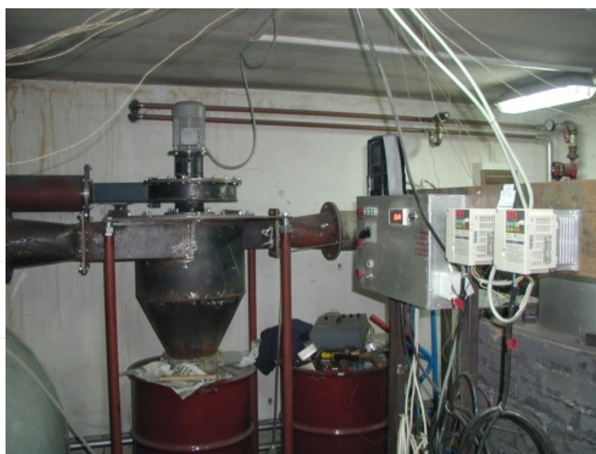
Figure 5. The boiler control system and cyclone-type particle precipitator
