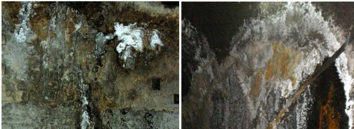
Fig. 1. Deterioration of railway tunnel (Southwestern Region, China)
