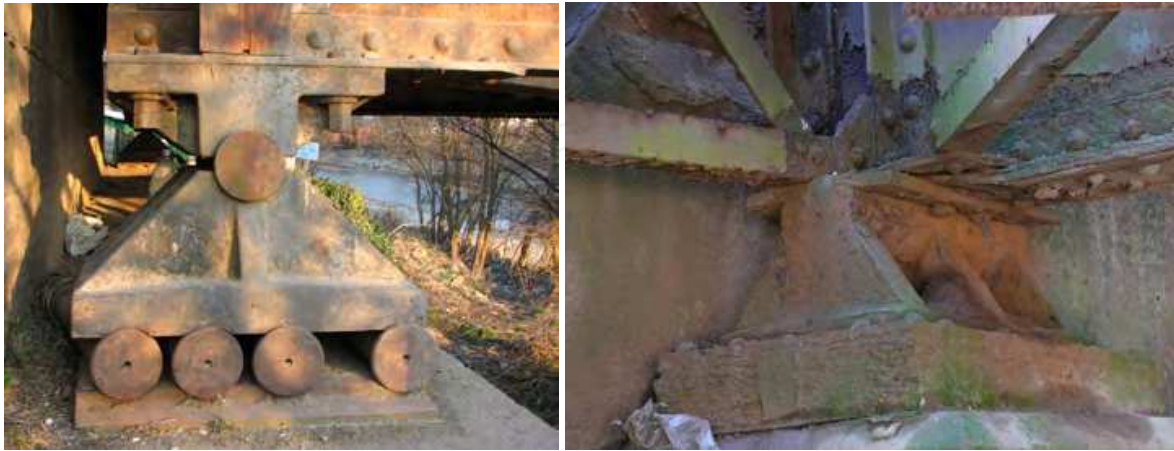
Fig. 5. Defects on bearings
