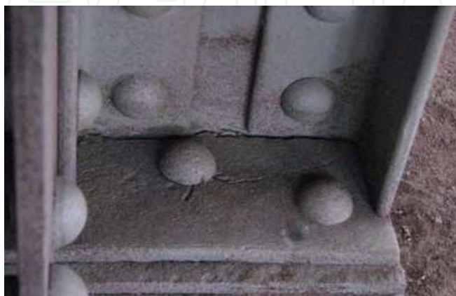
Fig. 4. Crack in the lower flange near to the bearing
