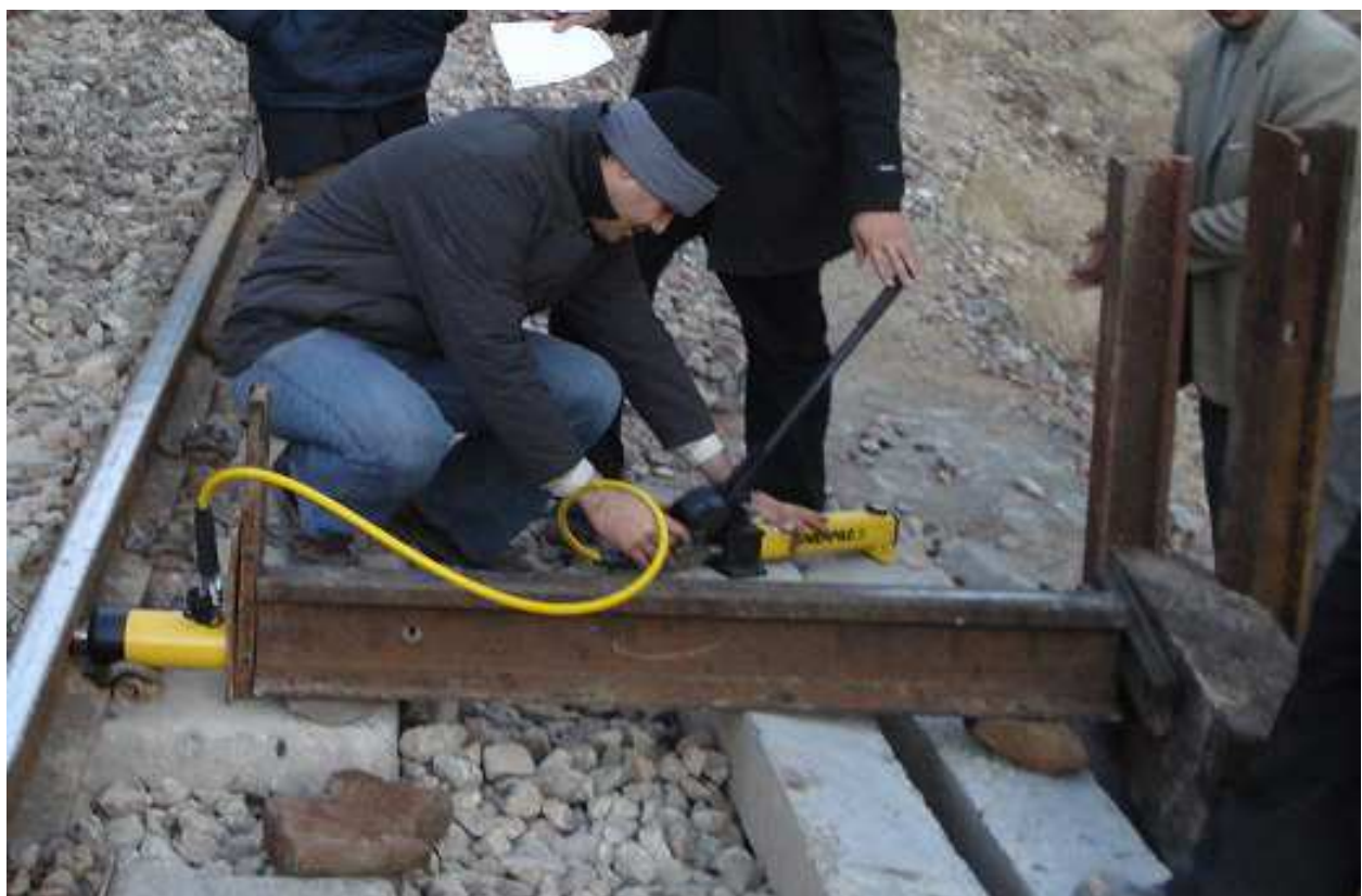
Fig. 15. Installation of the hydraulic jack
