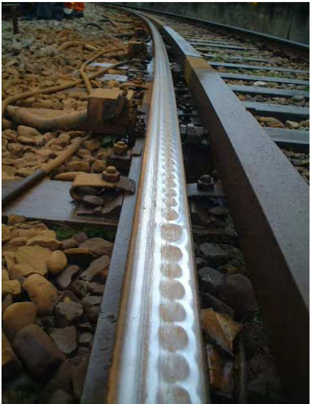
Fig. 2. Example of rail corrugation
