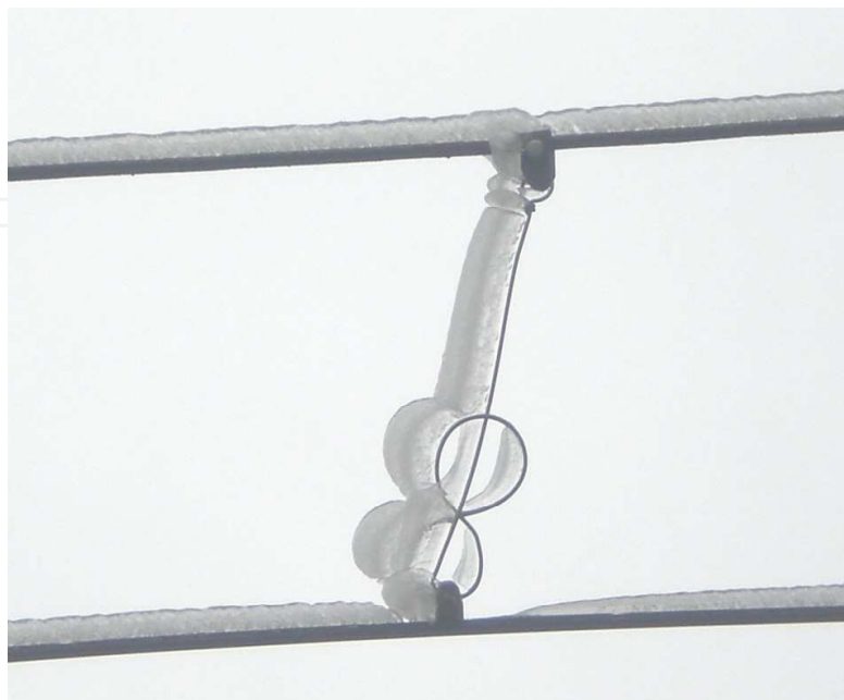
Fig. 2-2. Icing of contact wire
