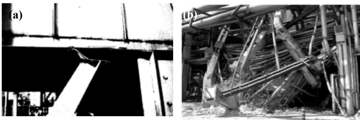
Fig. 7. (a) Damage to the supporting structure of fans (Loma Prieta, 1989), (b) Collapse of a piping system (Itzmit, 1999).
