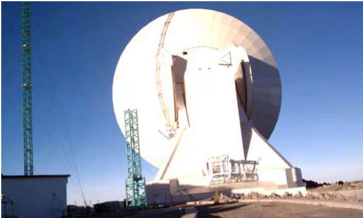
Fig. 6b. The GMT ( http://www.lmtgtm.org/images/sitepics05012011/LMTatSunrise1.jpg ) observatory construction site, with the last ring of the antenna in the process of installation.
