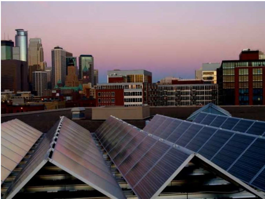
Fig. 4. Non-tracking LCPV design with 3M Cool Mirror (photo courtesy of Ray Colby with Sundial Solar). Peak power output increased by up to 60% as shown in Figure 5 with the use of 3M brand Cool Mirror 330 film in the reflector modules of the RAIS WAVE reflector design.
