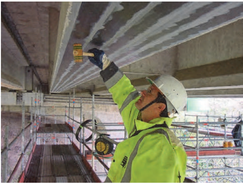
Fig. 1. Inspection with acoustic sounding (hammer tapping).
