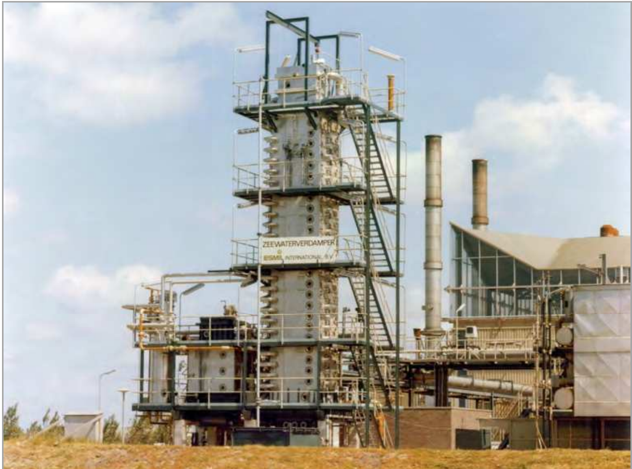
Fig. 11. MSF / FBE evaporator, Isle of Texel.
