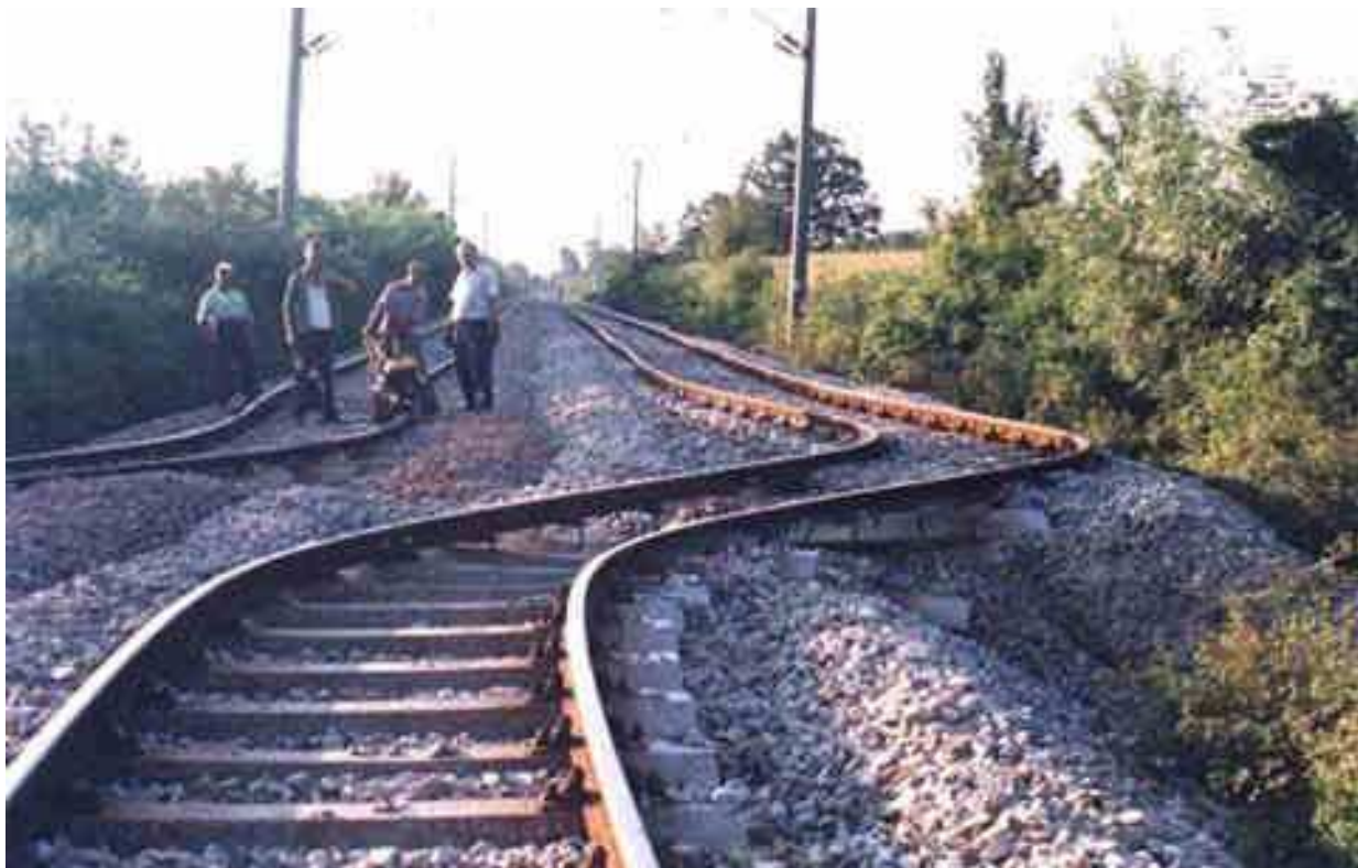
Fig. 9. An example of rail way which build on fault zone and is cutted by this zone in Turkey after 1999 Marmara Earthquake. It is taken from http://www.resimkarikatur.com/resim1684.html . Photographer is unknown.
