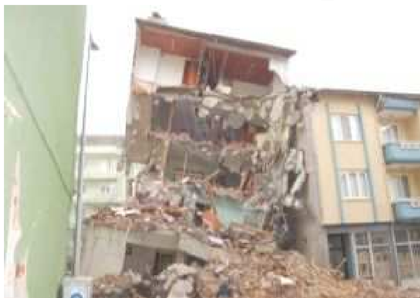
Fig. 10. An example of collapsed structure because of building design and different construction height after 1999 Marmara Earthquake. It is taken from http://www.haberingundemi.com/haber/Depremin-Simgesi-Bina-Yikildi/80399 . Photographer is unknown.
