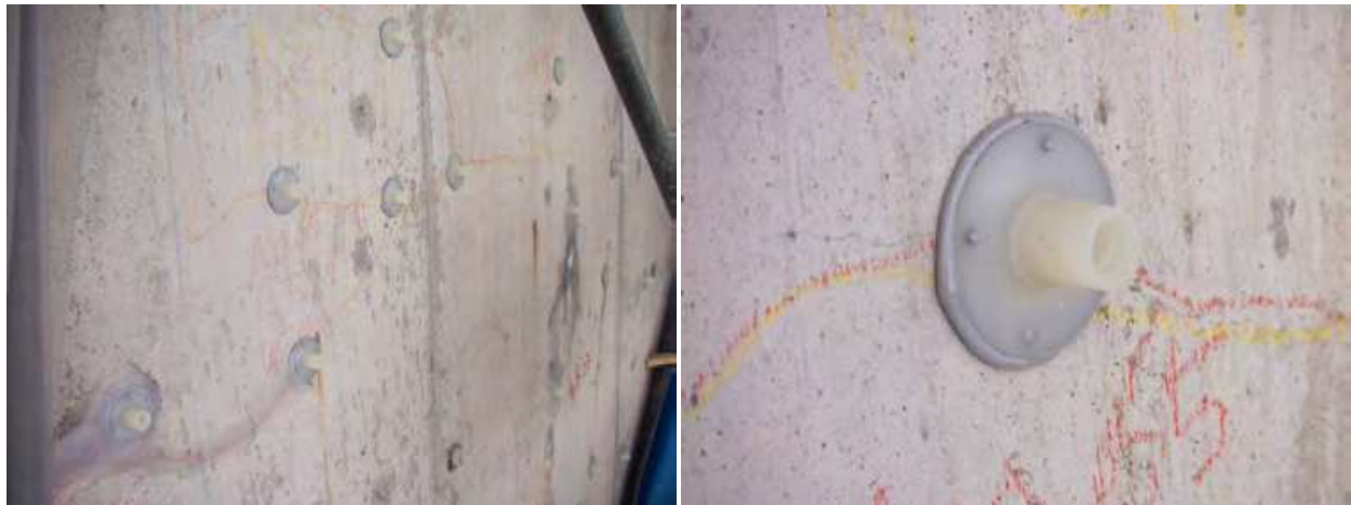
Fig. 1. (a) Multiple locations of injection on the surface, (b) detail of the injection point.
