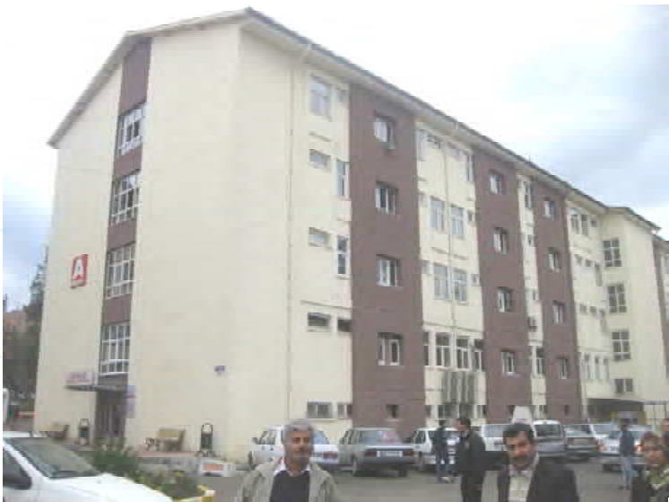
Fig. 8. An external shear wall strengthened building
