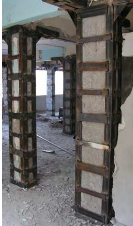
Fig. 13. Steel jacketing applied to RC columns (Photo by Dr. Ali Haydar Kayhan)
