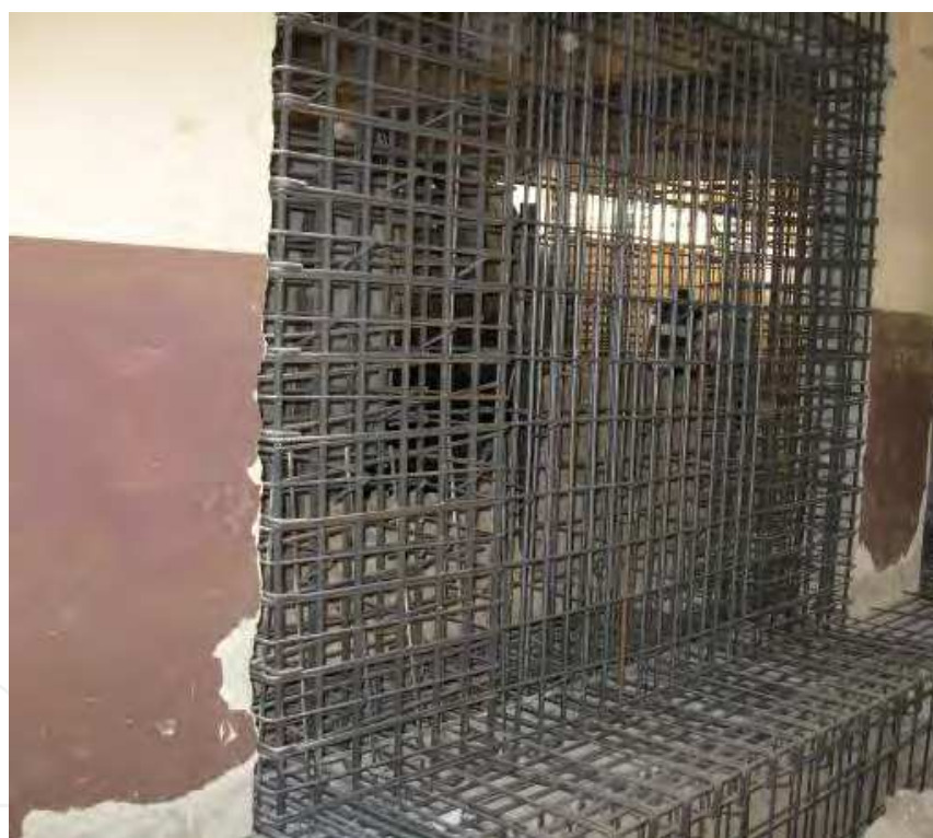
Fig. 3. Infill wall application in an RC building
