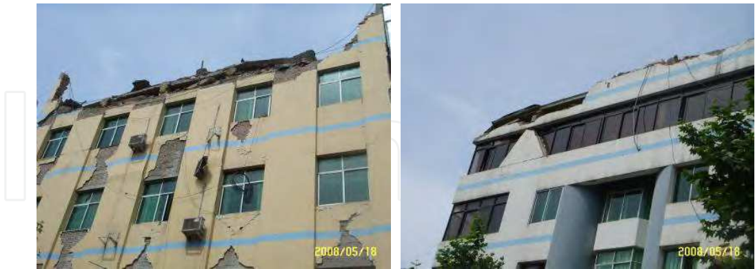
Fig. 4. Failure of the parapet wall
