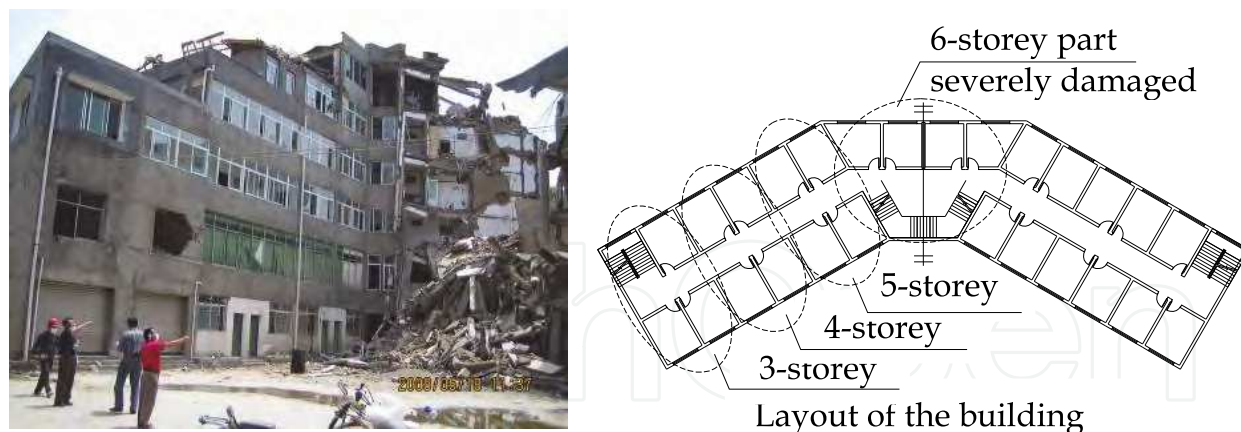
Fig. 7. Severe damage of masonry buildings with elevation irregularity
