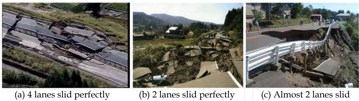
Photo 1. Large-scaled damage of road embankment without traffic performance
