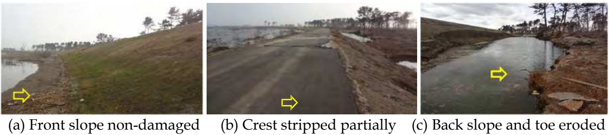
Photo 8. Dyke overflowed by tsunami
