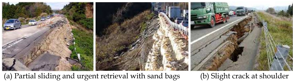
Photo 2. Small-scaled damage of road embankment with a certain traffic performance
