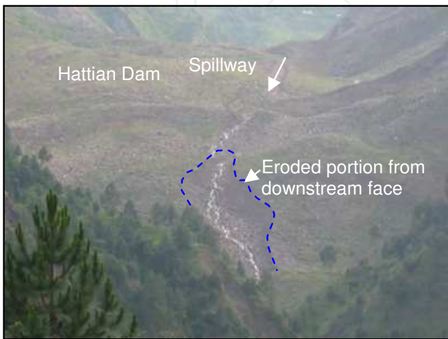
Fig. 7. Front view of the Hattian landslide mass, showing the downstream face erosion.
