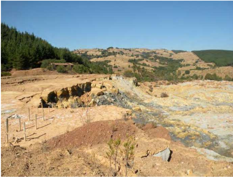
Fig. 24. Upper Scarp of Failed Tailings Impoundment. (GEER 2010)
