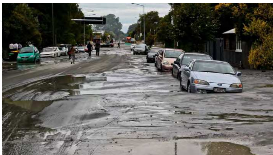
Fig. 26. Liquefied Sand Deposited on Street, 2011. http://otilya.com/view/ News/Asia-Pacific/New-Zealand
