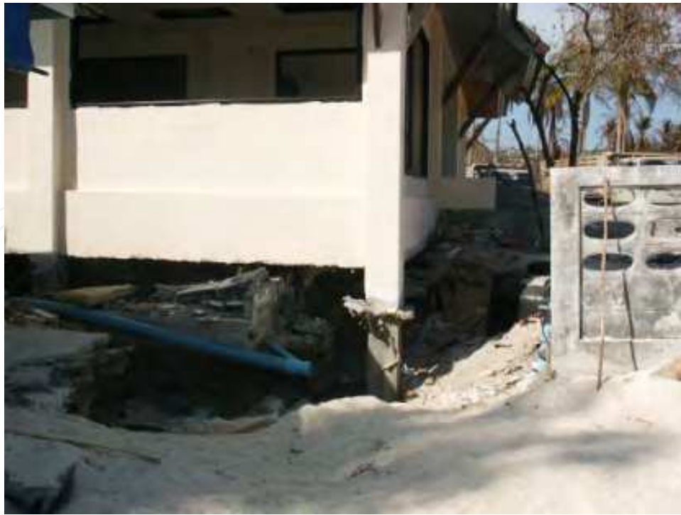
Fig. 40. Scouring of Foundation Soils and Severing of Building's Utility Lines, Phi Phi Island Hospital, Thailand, 2004.
