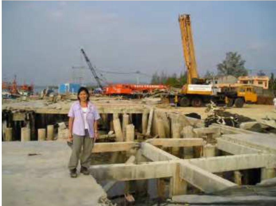
Fig. 36. Wharf Damaged by Wave Impact and Uplift, Bam Nam Kem, Phang Nga Province, Thailand, 2004.
