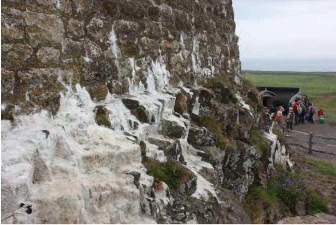
Fig. 1. Speleothem (flowstone) attributed to carbonate leaching from lime rich mortar, Lindisfarne Castle, Northumberland, UK.
