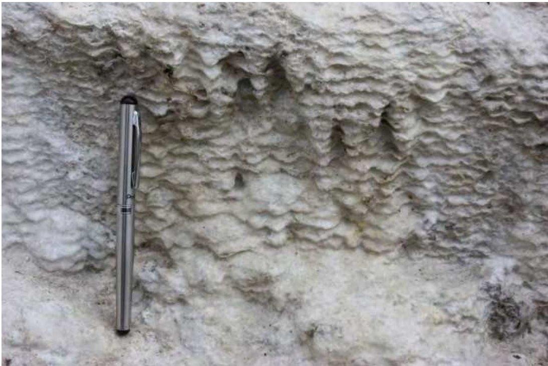
Fig. 2. Speleothem (flowstone) attributed to carbonate leaching from lime rich mortar, Lindisfarne Castle, Northumberland, UK.
