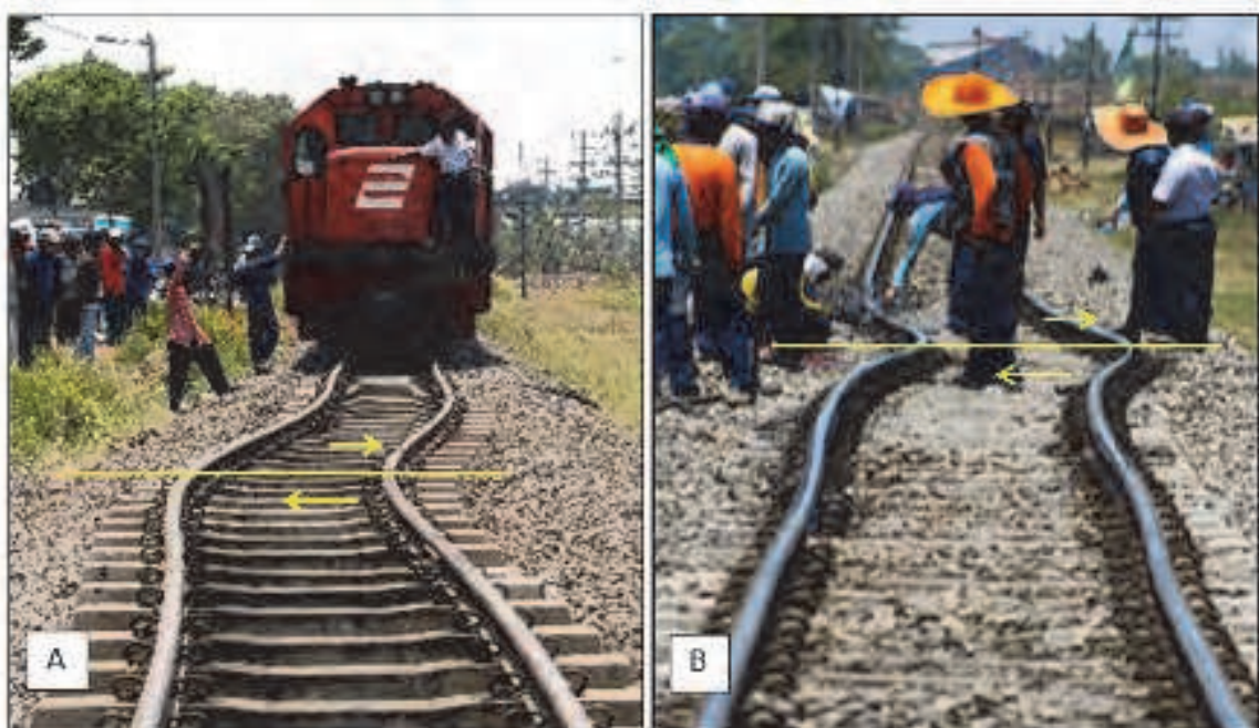
Fig. 11. Shear stress have damaged nearby infrastructures such as the dextral movements of a railway, bursting of a gas pipeline and numerous breakages of water pipelines at the same location further supports displacements along faults. (A) The railway bent to the west of main vent on September 2006. Offsets that occurred approximately 40 cm with orientation direction NW - SE. (B) At the same location, the railway was bent again in October 2009, with an offset of approximately 45 cm. The bending of the railway line is due to fault reactivation that often has differential movements which created shear stress.
