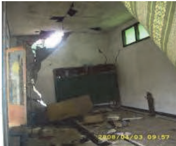
Fig. 29. A mosque located in the Renokenongo village, to the east main of the vent is damaged due to fault reactivation. At this location a lot of fractures were oriented NE-SW, and these are patterns of the Watukosek fault system.
