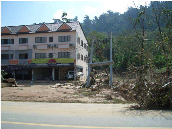
Photo 4. Electric pole tilted as a result of the scouring of the ground by the tsunami (Khao Lak, Thailand)
