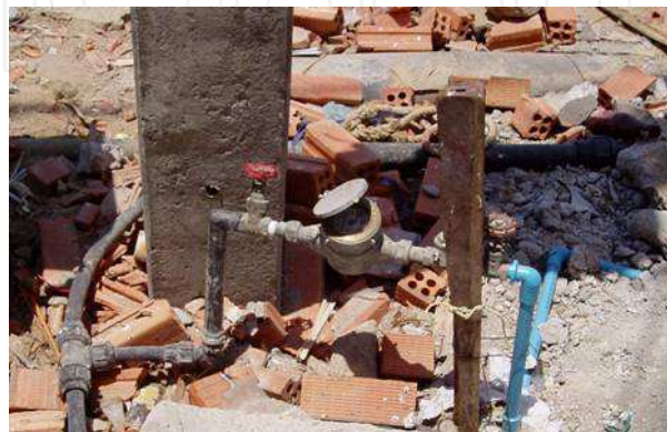
Photo 2. Water meter above ground. Black-colored polyethylene pipe is the service pipe of PWWA, and the blue-colored vinyl pipe is the residential pipe (Khao Lak, Thailand)
