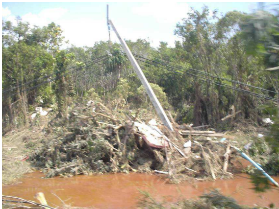
Photo 3. Electric pole tilted by collision with tsunami driftwood (Khao Lak, Thailand)
