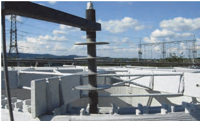
Fig. 3.1.6. One of the four sensors installed on the top of the coil.
