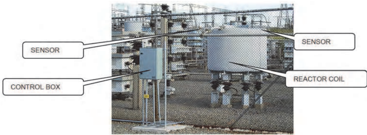
Fig. 3.1.7. The reactor coil and the sensors installed.
