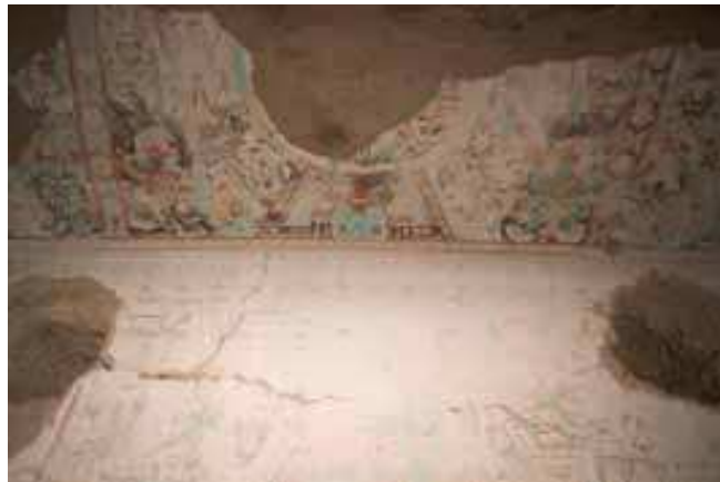
Fig. 1. Delaminated wall paintings in Cave 329 of Mogao Grottoes
