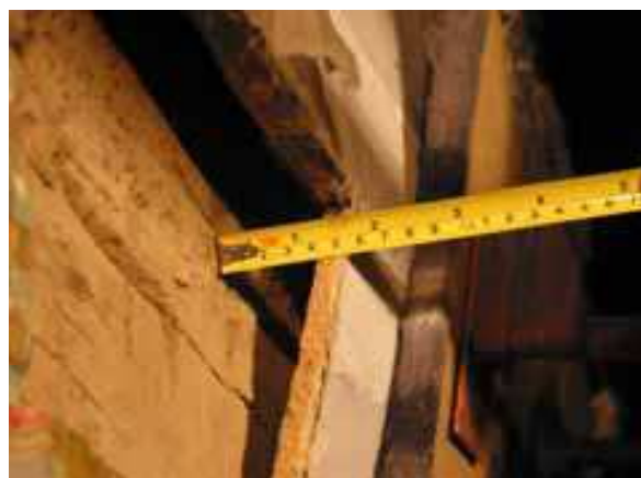
Fig. 2. Delaminated wall paintings in Eastern Audience Hall of Potala Palace
