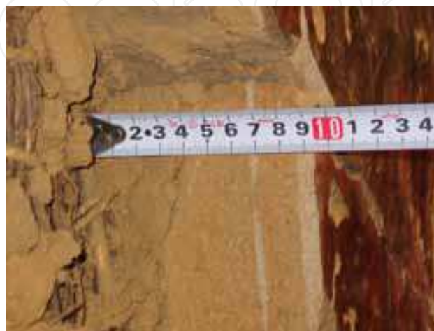
Fig. 3. Typical plaster section of wall paintings in Potala Palace
